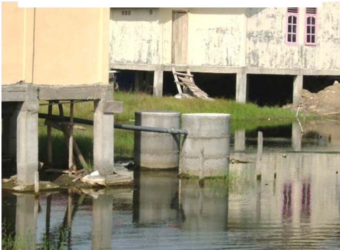
Exposed waste piping & septic tanks (actually leach-pits) in very high water table (Meuraksa, Banda Aceh) Master Plan by SOGREAH for BRR
