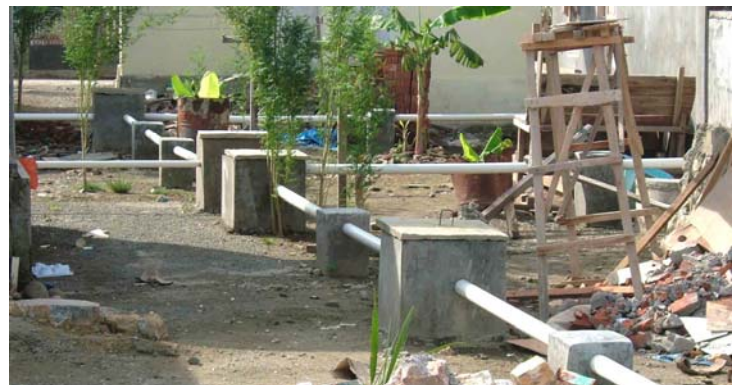
Exposed wastewater piping to public drains. Drains act as open sewers. Drains have no slope, wastewater breeds flies, mosquitoes & pathogens
