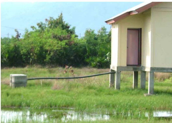
Exposed wastewater piping to public drains. Drains act as open sewers. Drains have no slope, wastewater breeds flies, mosquitoes & pathogens
