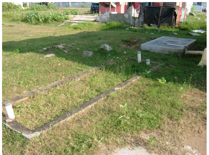
3 PICS ABOVE Canadian & American Red Cross Poorly constructed wetlands with no plants (Kahju, Aceh Besar)
