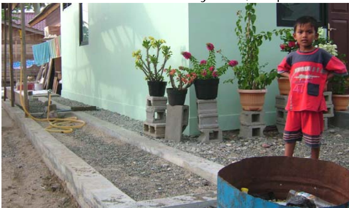
ARC ARC/BRCS Wetland system, no plants
