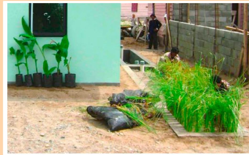
Tertiary Treatment and Disposal 10m x 1m Vegetated Leachfield
