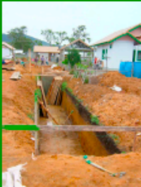
excavation 30m long
