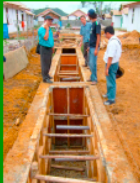
formwork & piping
